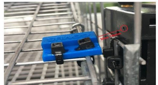
The distance between the magnet and the small hole in the bracket must be less than 10mm.
